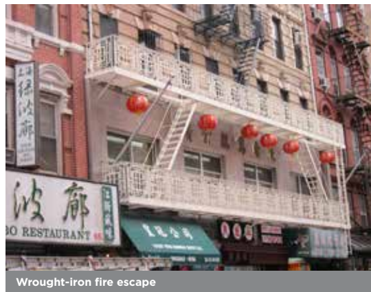
Wrought-iron fire escape
