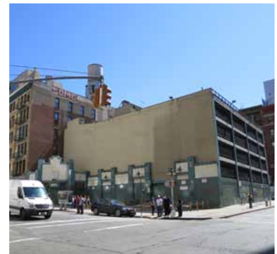
Potential redevelopment of 2 Howard Street for cultural uses, including a movie theater.
