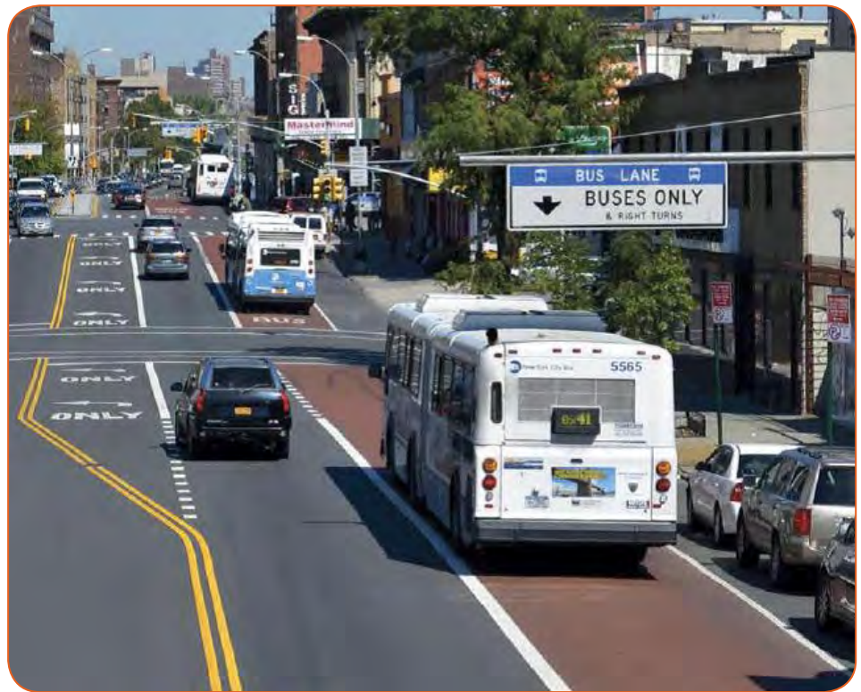
Bx41 Select Bus Service on Webster Avenue – parking and loading space maintained
