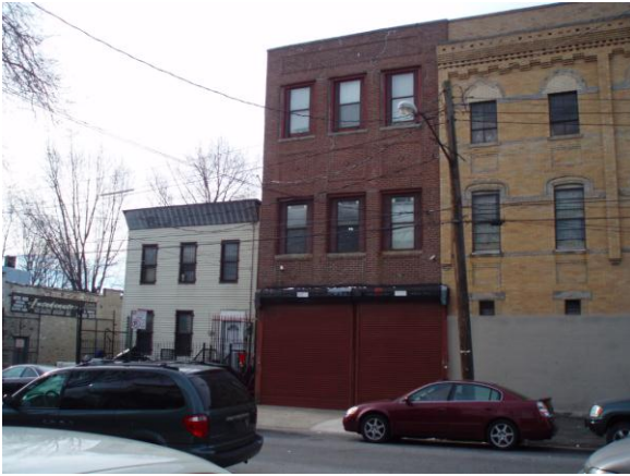
Caption: 26 Milford Street (red brick building)
