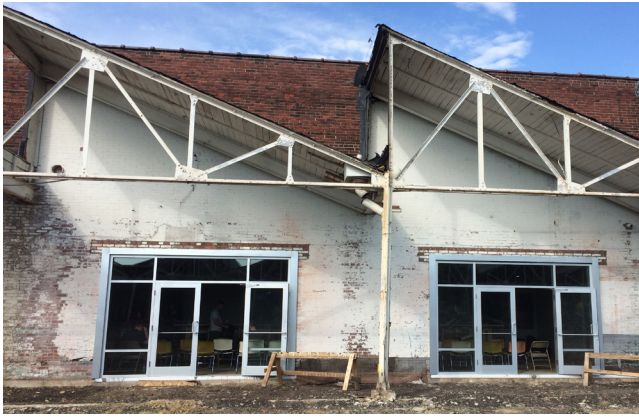
Centerpoint Brewing is currently developing a 30-barrel brewing system in a 17,500 square foot space in the Circle City Industrial Complex, set to open in early fall 2016.
